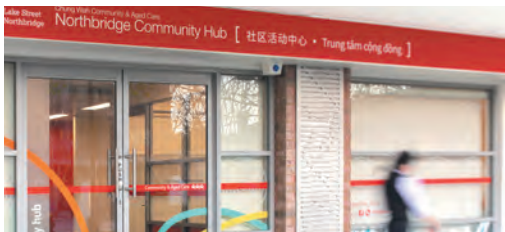
Chung Wah Community & Aged Care NORTHBRIDGE COMMUNITY HUB 2/98 Lake St, Northbridge
